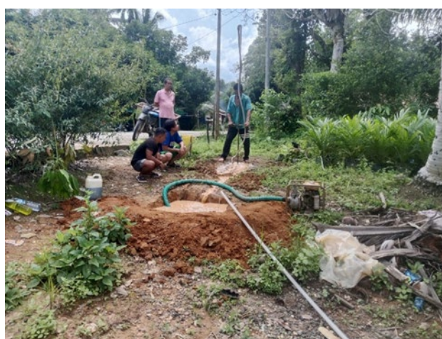
Figure 2. Construction of bore wells per neighborhood unit (RT)
