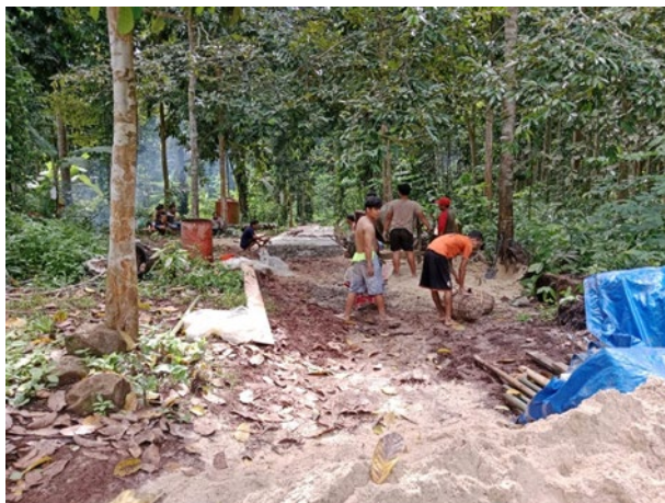
Figure 1. Construction of farm access roads
