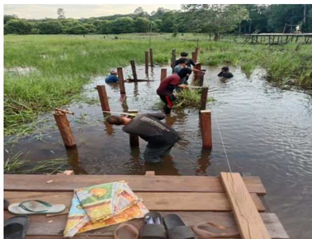
Figure 3. Construction of an ironwood bridge in a rice field area
